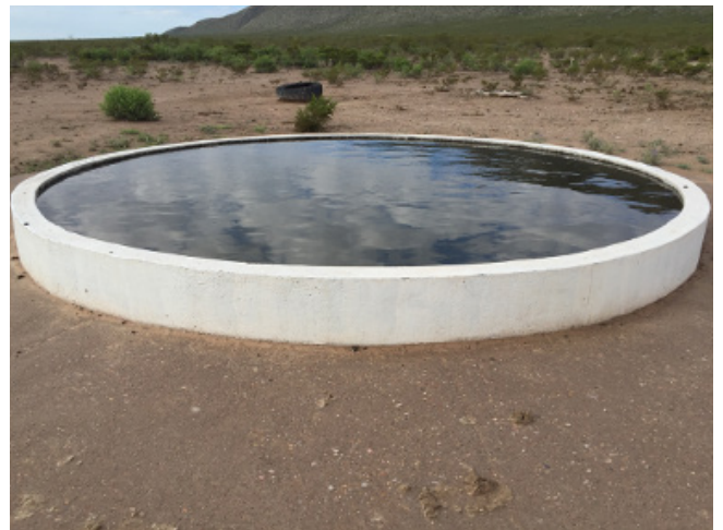
Circular Trough (2,500 gallons).
